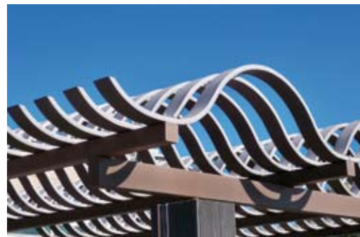
ceiling constr. installed 2003 - timeless beauty
